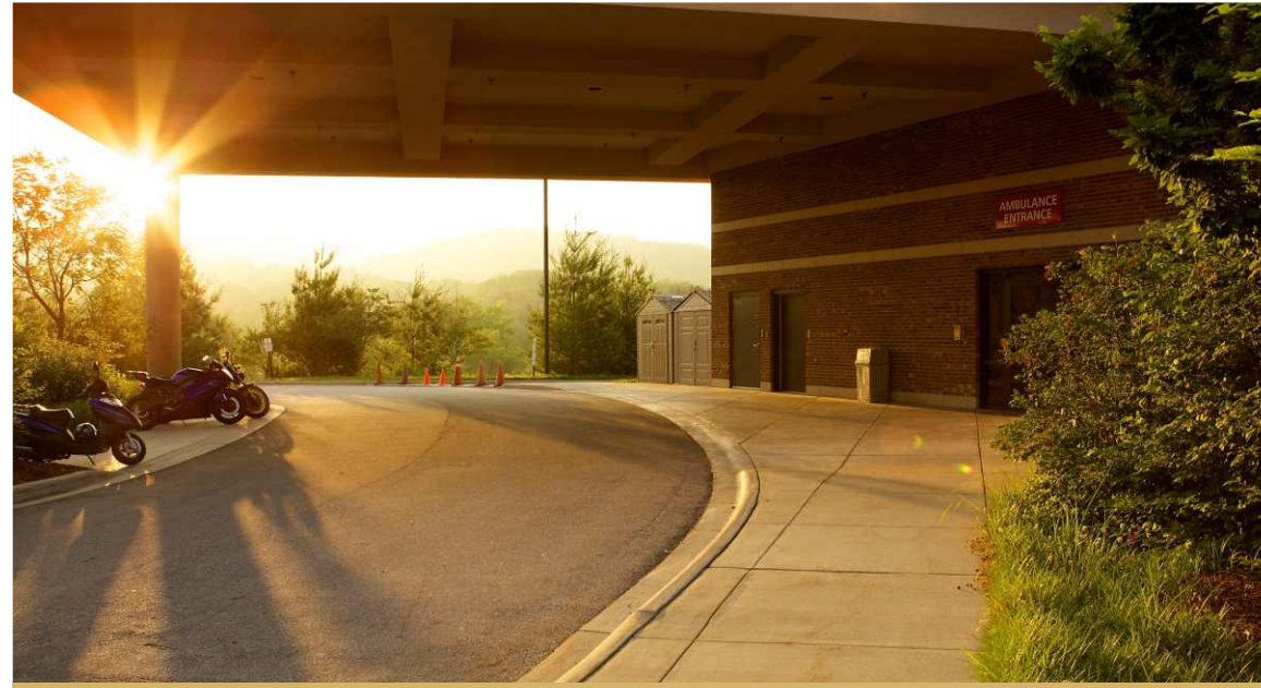
WIDE ROADS ENCOURAGING NATURAL VENTILATION
